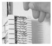
8. Use the bridging clips to connect the middle metal clips if necessary.
