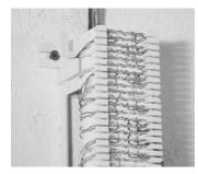
5. Route each pair through the same slot in the strip. Separate the conductors of each pair and place them in the appropriate metal clips.
