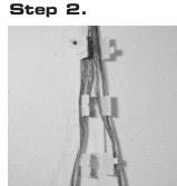
2. Route the horizontal or backbone cables inside the 89B mounting bracket and feed the cables out either side of the bracket.
