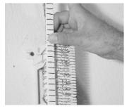
7. Install the labeling strips (not included) and label each station as necessary.
