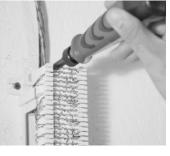
6. Terminate each conductor by using the 66 single blade punch-down tool.
