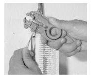
4. Use the UTP cable stripper tool to strip back cable jacket as close to the termination point as possible.
