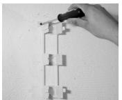
1. Mount an 89B mounting bracket (sold separately) on a plywood wall by using two wood screws.
